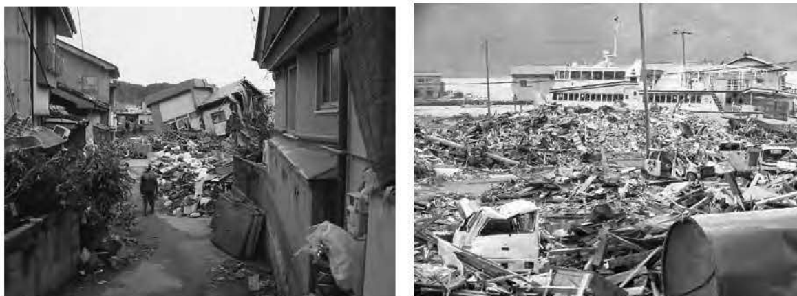
[宮古市内の被害の様子]
